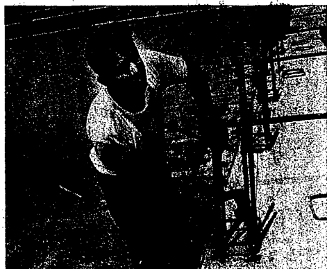
MILT COTTRELL, of Livonia, works on the overpasses along the Jeffries Freeway. A steelworker, he lays the steel rod foundation over which cement is poured. Here he is straightening wires which are used to support the overpass. (Observer photo by Bob Woodring)
