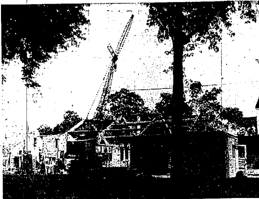
WORK IS PROGRESSING rapidly on the new First Baptist Church addition being constructed on Shiawassee at Farmington Road adjacent to the present church building. Last week workmen began putting up trusses in preparation to the overhead enclosure of the building. A large crane can be seen in the photo lowering another truss into place.
