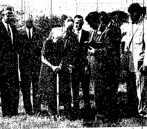
TURNING THE FIRST shovel of dirt at ground breaking ceremonies of the new North Farmington Baptist Church on 13 mile Road a week ago Sunday.
