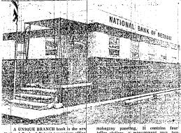
A UNQUE BRANCH bank is the new National Bank of Detroit temporary office open recently a 33200 Twelve Mile, near Parmington Road. The office is tinusual in that it is made up of two 10-foot by 36-foot custom built trailers which have had the wheels and adjoining partitions removed and are botted together and secured to a foundation. The unit is insulated and finished in
