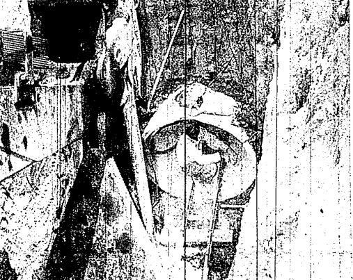
FIRST PIPE in the multi-million dollar Farmington interceptor sewer system was lowered into the bottom of this 19-foot trench. The work was started on the north side of Nine Mile road, and the pipe will be pushed under the roadway to the south side, thence laid the remainder of the way to the south end at Shiawassee.
