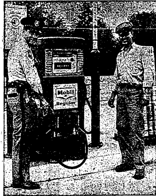
ROUTINE CHECK of a gasoline pump at the William Taylor station, 37885 Ann Arbor Trail, by Corp. William Crayk, of the Livonia Police Department's Weight and Measures division, is saving Taylor a lot of money these days. Corp. Crayk discovered Taylor's pump has been giving 11 gallons of gas while registering 10. It didn't take Taylor long to have the pumps repaired to deliver 10 gallons for 10 on the meter.
