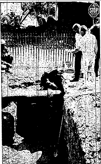
IT TOOK 37 MINUTES for a crew to install an eight-inch water main from the Plymouth system to the Haller Manufacturing Plant on Northville Road last Saturday. The plant was without water only a few minutes during the endeavor, thanks to the co-operation of the Plymouth Township and City Fire Departments. DPW Supt. Joseph Bida is shown watching workers making the final connection — water flowed through the main within minutes.
