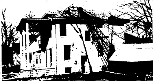
THE OLD THAYER FUNERAL HOME on Grand River at Grove Street went under the wrecker's ball last week to make way for a new building to house the new Goodyear Tire Company outlet in Farmington. The Thayer Funeral Home moved into new
