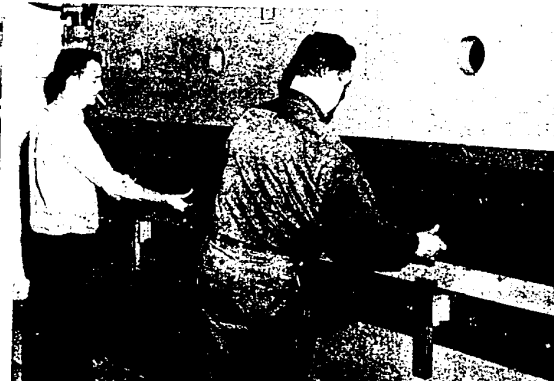
A MACHINE THAT CAN BEND one-quarter-inch sheets of steel is in operation (above) at Diamond Automation. Two workmen are shown making the second right-angle bend in the material.
