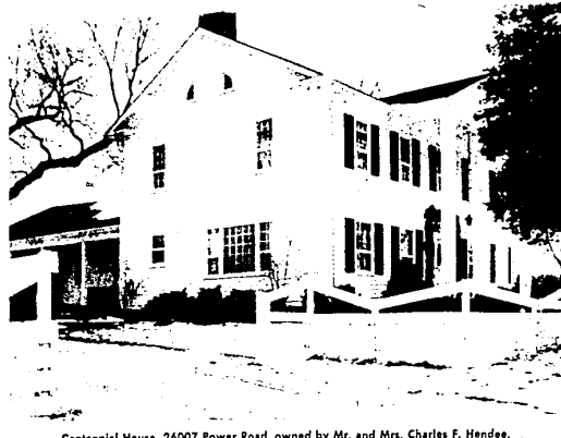
Centennial House, 26007 Power Road, owned by Mr. and Mrs. Charles F. Hendee.
