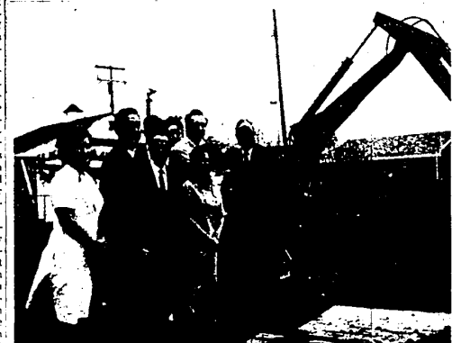
THE SHOVEL on the scene marks the official ground breaking of the new civic center in Farmington. (Left to right) Mrs. Johnston, Danny Pevos, Dr. Ira Altshuler, Sharon Agee, Mrs. Weisman, Dr. Weissman (with foot on shovel) assisted by Livonia Council President Peter Ventura.
