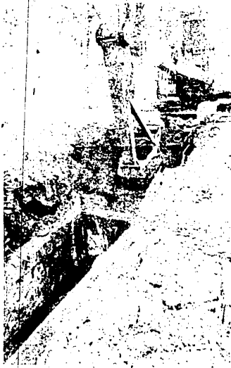
CONSTRUCTION --New sewer and water lines have been installed throughout the township. Here the machine digs a trench for the installation of water lines in the southeast section of the township.
