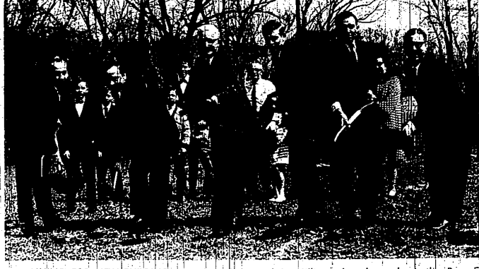
AIMING FOR NEW BUILDING — Leaders of the Trinity Assembly of God in Farmington turned the first shovel of earth Sunday as ground was broken for a new building. From left are D. Mobat and R. Milligan, board members; the Rev. E. Cooley, Assembly of God district superintendent; the Rev. A. Worthley, assistant pastor; T. Mason, board member and the Rev. John Winn, pastor.
