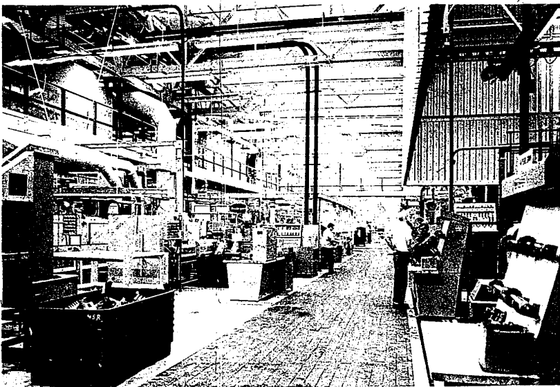
QUIET. That's how the new Cadillac-Livonia plant impressed Observer Roving Editor W. W. Edgar, who noted that the interior is soundproofed and engine blocks slide along the assembly line so quietly that one hardly notices them.
